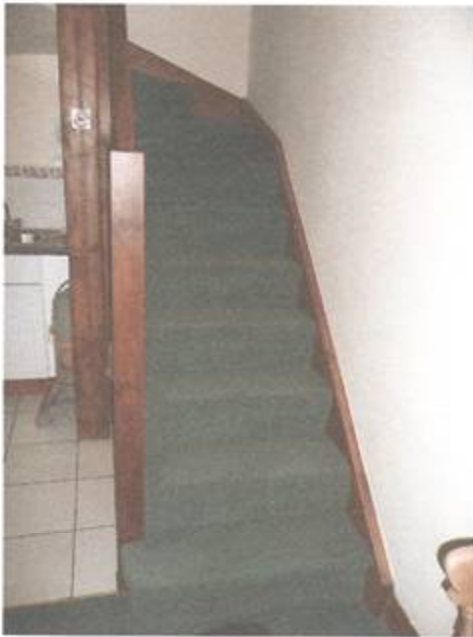
There are 13 stairs from the ground floor to the 1 st floor the height of each step is 190mm
