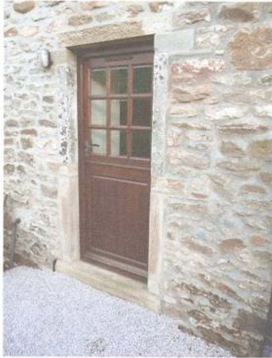
Door 2 is 800mm wide and there is 1 step, the height of which is 130mm
