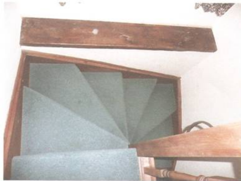
There are 13 stairs from the ground floor to the 1 st floor the height of each step is 190mm
