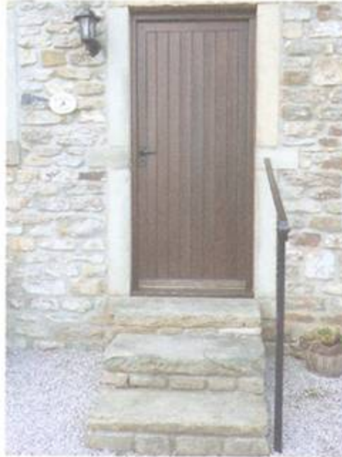
Demdyke Cottage door 1 835mm wide There are 3steps to the front of this door Step 1 180mm high Step 2 200mm high Step3 150mm high
